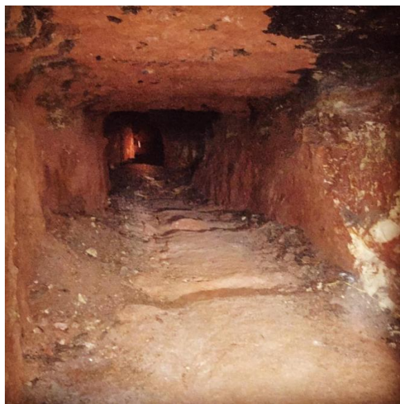
Adit or drive through the laterite. The shallow cross trenches would have held wooden sleepers that the rail track was laid on
